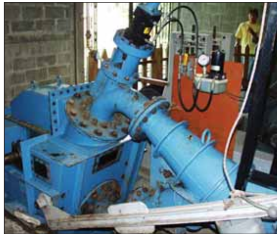
(b) A 230 kW mini-hydro scheme for village electrification in upland Nicaragua.
