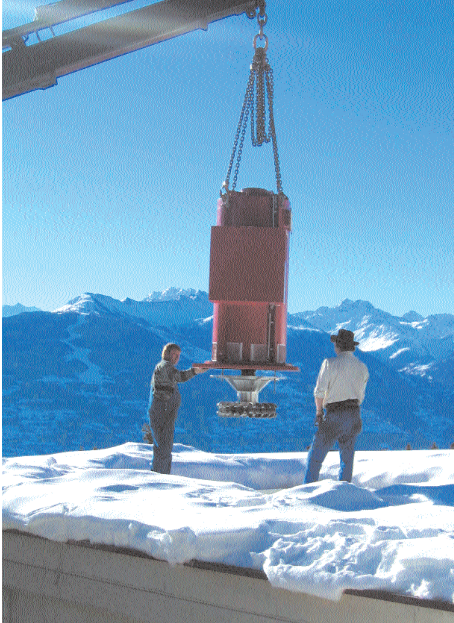
Installing a small hydro turbine in the mountains of Switzerland MHYLAB
