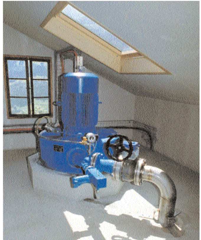
The turbine in the Troistorrents drinking water system MHYLAB
